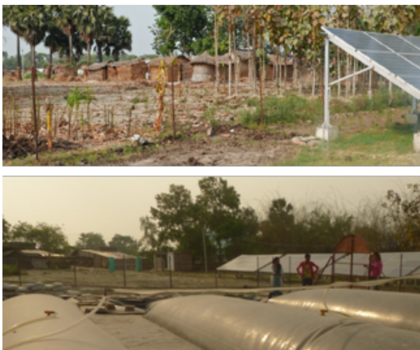
Figure 2. Combined solar –biogas installation at Beldi, Bihar (State of Bihar, Images sources: J. David Tàbara, April 2017).
