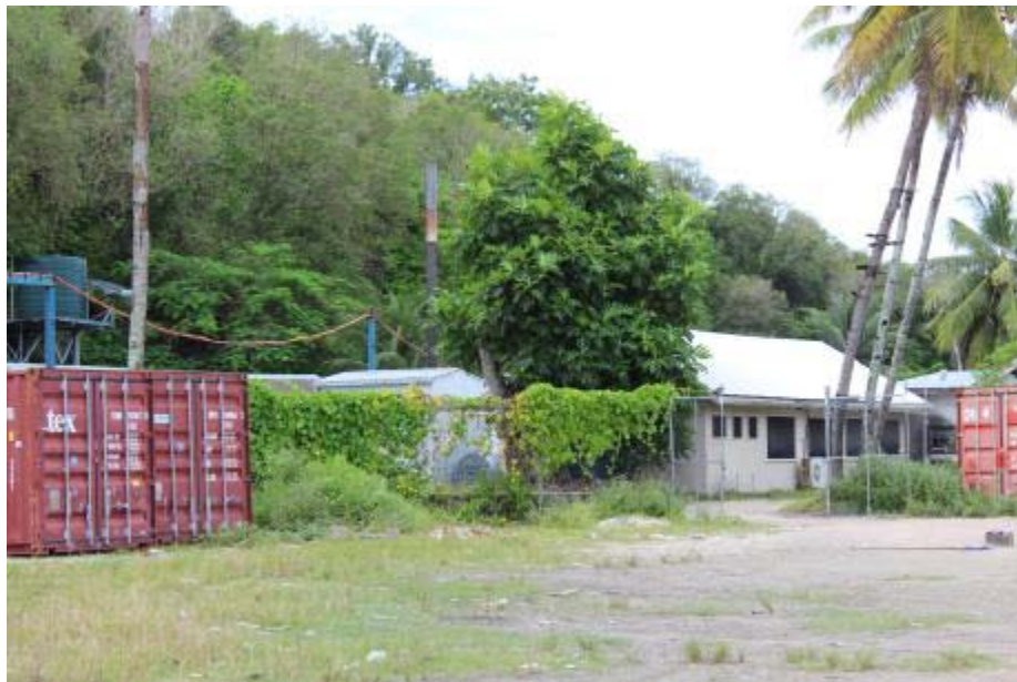
Photo 8: Location of the incinerator at the Hospital (taken 11/0/42014 by Trevor Thornton)
