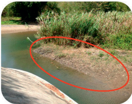
Figure 6.5. Siltation within the dam due to sediment trapping
