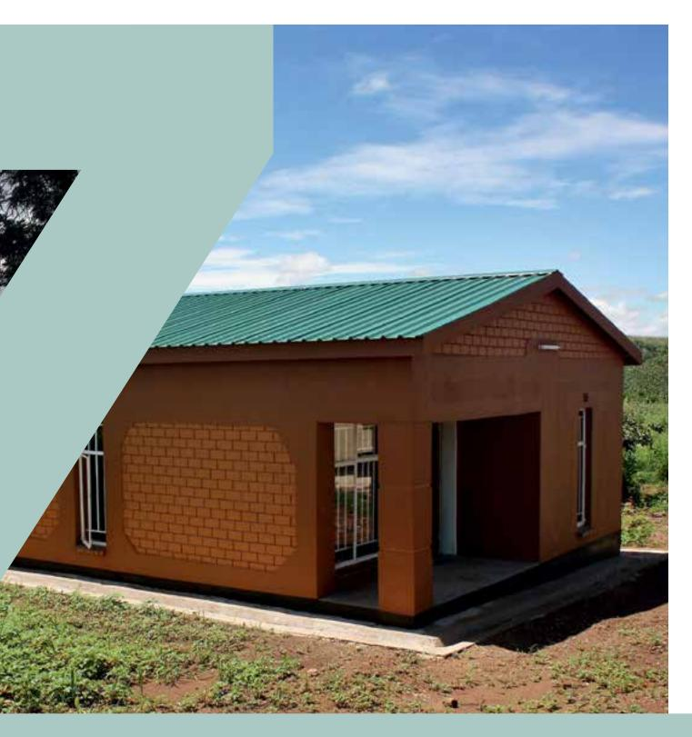
Developing Zambia's Sustainable Housing Guidelines meant eight houses were built to test and demonstrate ways of incorporating sustainable principles in the construction of homes. These "pilot houses" prove that comfortable and affordable homes can be built while prioritising locally sourced, unconventional building materials and boosting the local construction sector.
