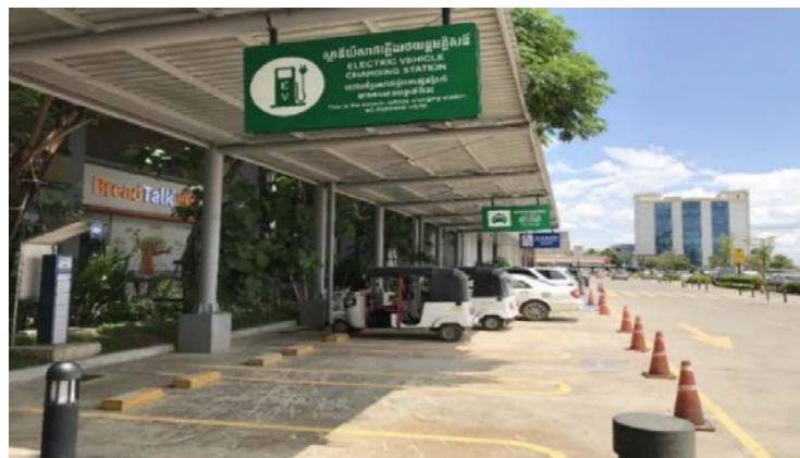
Figure 22. EV Charging Station at a parking lot in a mall in Phnom Penh
