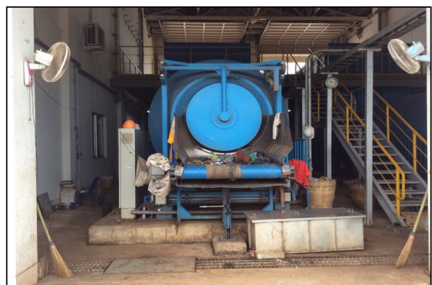
Loading and reloading point at the transfer station
