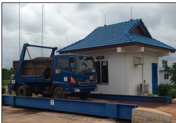
Weighbridge at the transfer station
