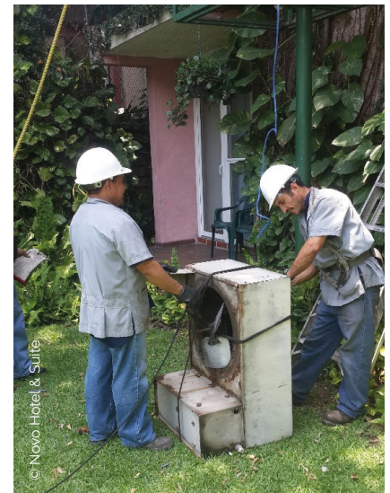
Installation of new air conditioners in Novo Hotel & Suite
