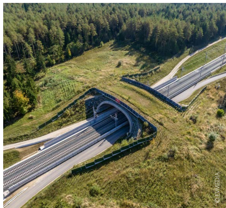
CONCRETE SHELL GREEN BRIDGE IN THE DOBROWA FOREST
