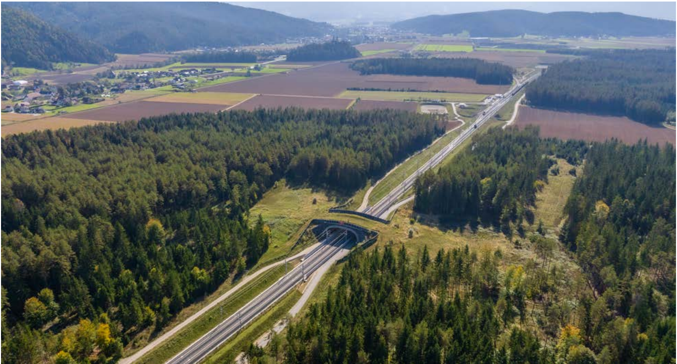
FIGURE 4 ARIEL VIEW OF THE KORALMBAHN GREEN BRIDGE, READY TO TAKE ON ITS ECOLOGICAL FUNCTION
