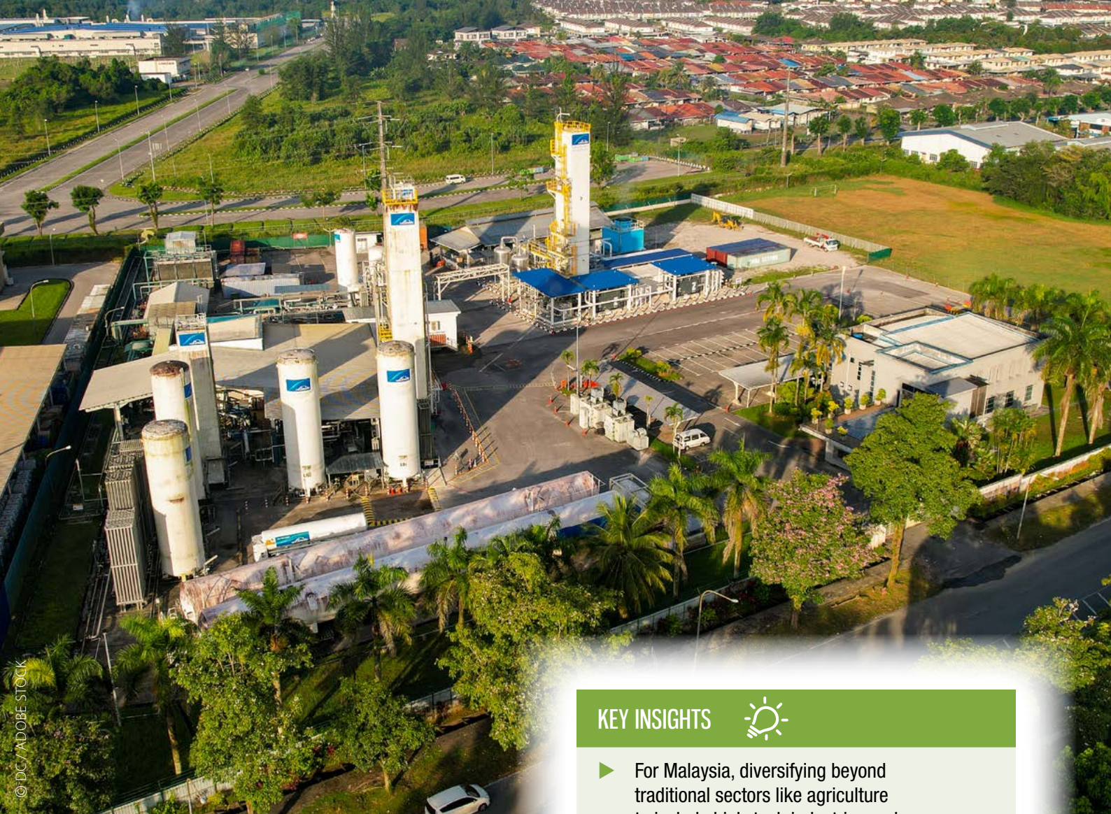
SAMAJAYA LIGHT INDUSTRIAL ZONE WHERE ALL THE MAJOR ELECTRONICS, SOLAR AND SEMICONDUCTOR PLANTS ARE LOCATED, KUCHING, SARAWAK MALAYSIA
