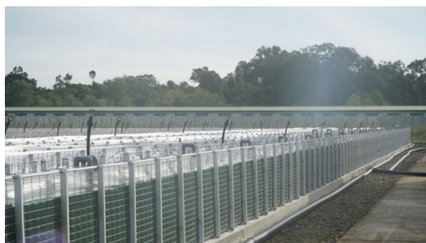
A microalgae cultivation facility utilizing photobioreactors, Brunei Darussalam
