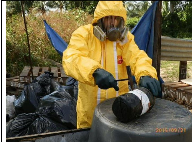
Figure 20: Container Puncturing to Prohibit Re-Use
