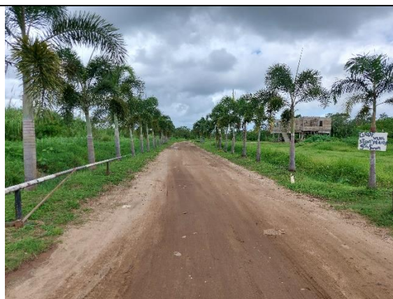
Appendix Figure 9.9-2: Entrance Road (Landfill Site North of Paramaribo)
