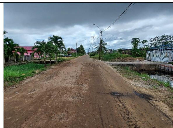
Appendix Figure 9.9-1: Entrance Road (Landfill Site North of Paramaribo)
