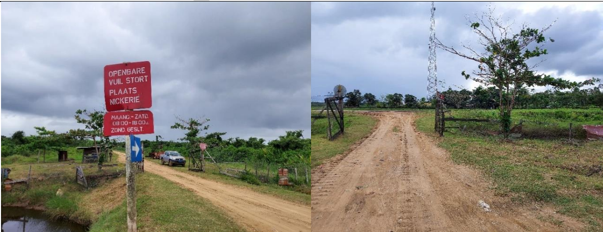
Appendix Figure 9.9-28: Entrance Road (Second Landfill Site Nickerie)
