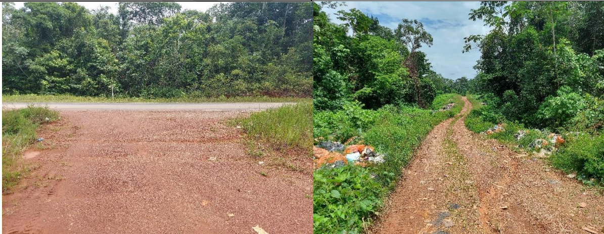
Appendix Figure 9.9-13: Entrance Road (Landfill Site Brokopondo)
