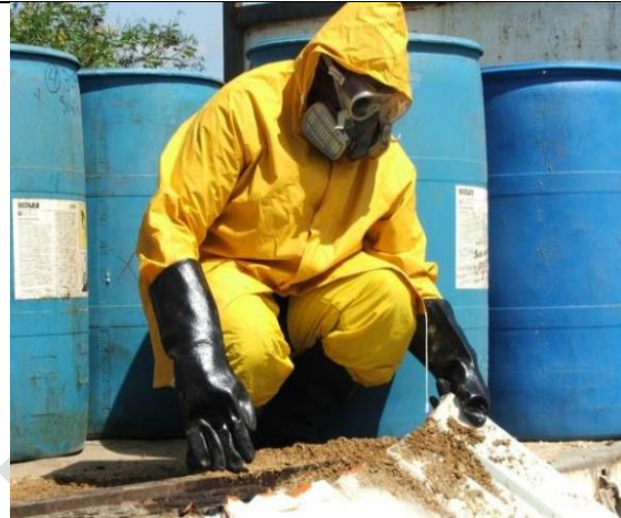
Figure 21: Personnel Preparing the Discharge Ramp
