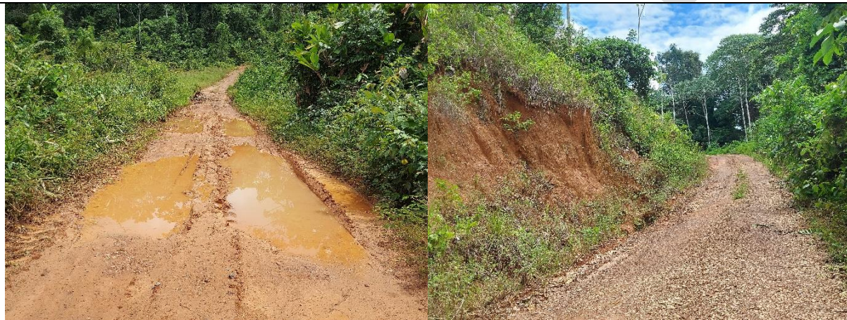
Appendix Figure 9.9-9: Entrance Road (Landfill Site for Sipaliwini)
