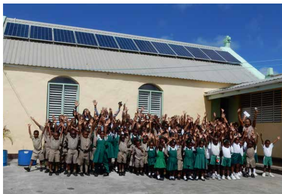
Solar panels installed on the roof of a school, Barbados
