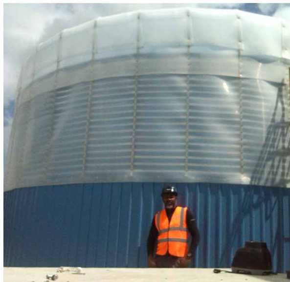
Biogas digester while under construction
