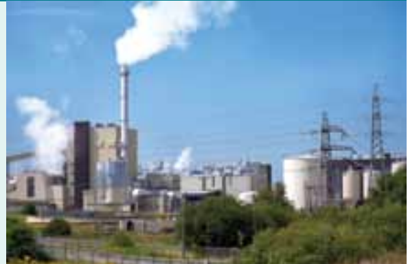
Shotton paper mill is saving CO 2 with a biomass Combined Heat and Power plant
