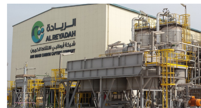
Al Reyadah carbon capture facility in Musaffah, Abu Dhabi Source: Masdar
