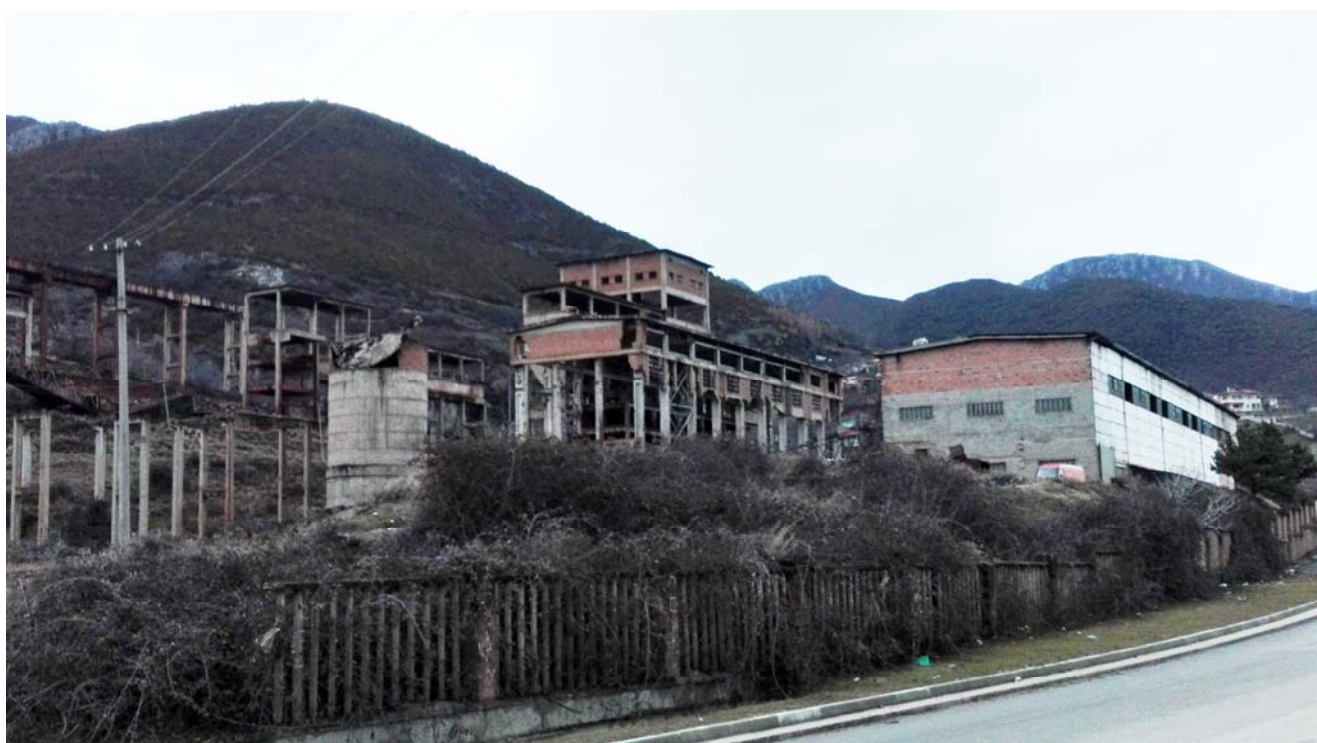
Photo 11.1: Abandoned site near Lake Ohrid
