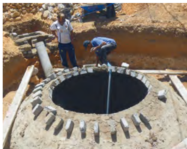
Morocco: constructing a biogas reactor for toilet waste and manure
