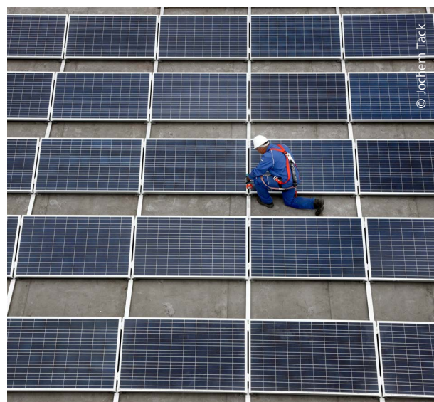
The CAM sub-region has high potential for RES development, including solar power generation.
