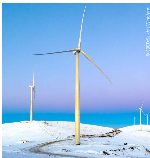
Salkhit wind farm generates approximately 5 percent of Mongolia’s electricity. However, there is
