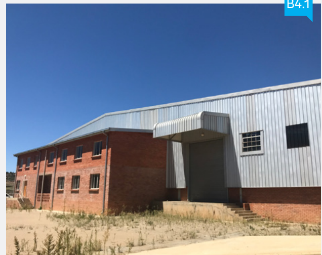
PHOTO B4.1. MARKET CENTER IN HA TIKOE
