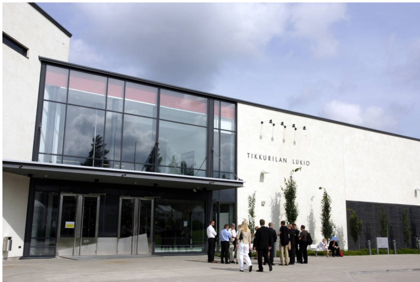
Figure 6: The main entrance of the Tikkurila Upper Secondary School, Vantaa, Finland
