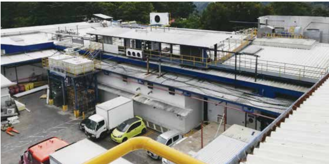
GENERAL VIEW OF THE FACTORY FROM THE PLATFORM WHERE THE EQUIPMENT WILL BE INSTALLED. PHOTO CREDIT: RODOLFO ELIZONDO
