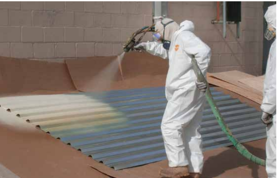
SPRAY FOAM TESTING AT URETHANE SYSTEM HOUSE IN MEXICO. PHOTO CREDIT: HORACIO HERNÁNDEZ DEL CASTILLO
