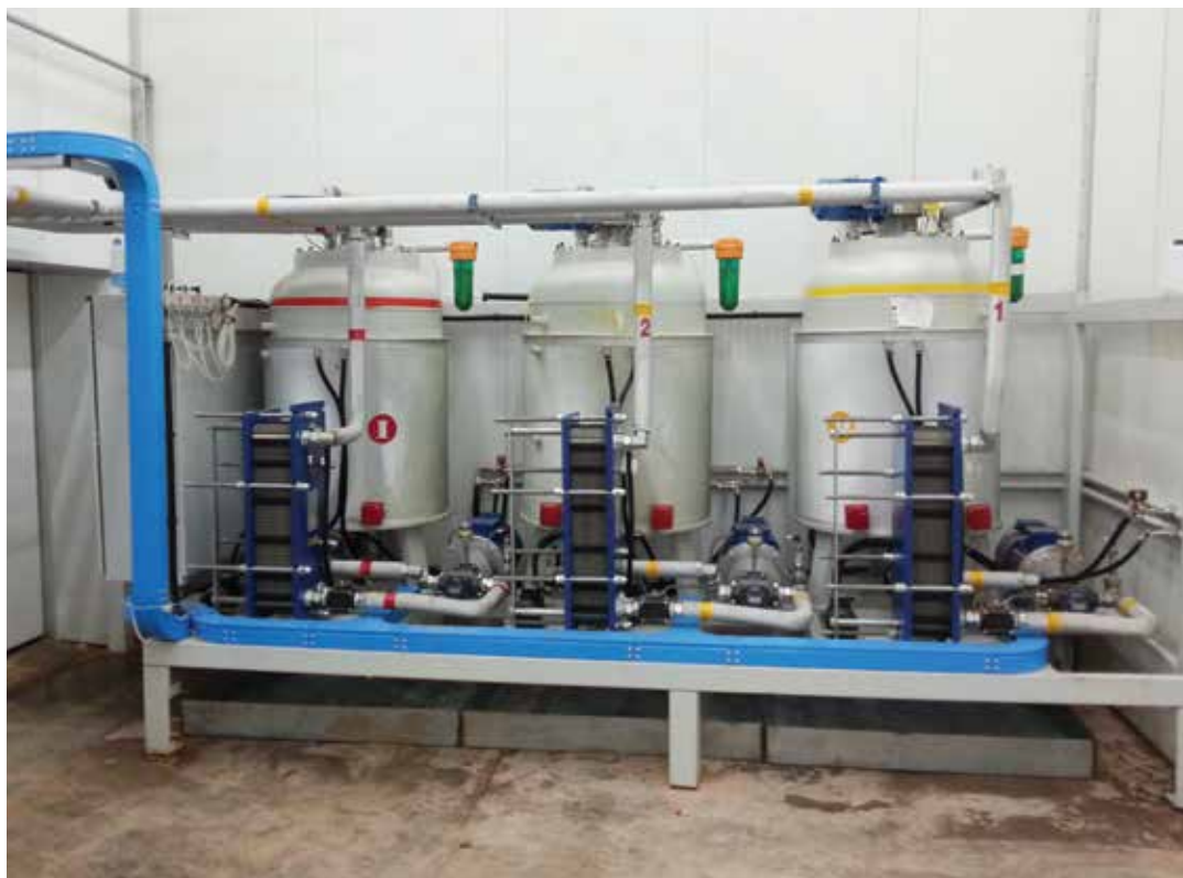
USE OF PENTANE IN FOAMING OPERATIONS AT REFRUCK COMPANY, EGYPT. PHOTO CREDIT: THE PROJECT TEAM
