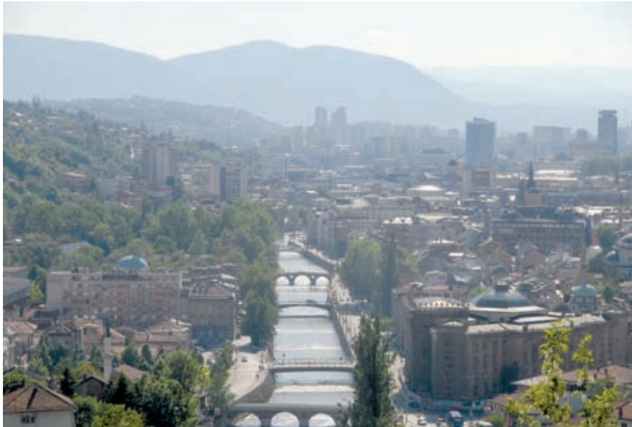
Photo 1.1: Miljacka River in Sarajevo
