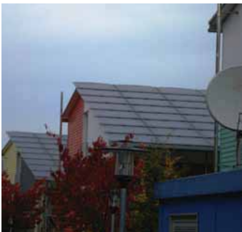
Solar PV panels on the rooftops of the "energy plus" houses © Gabriela Weber de Moraes, 2009
