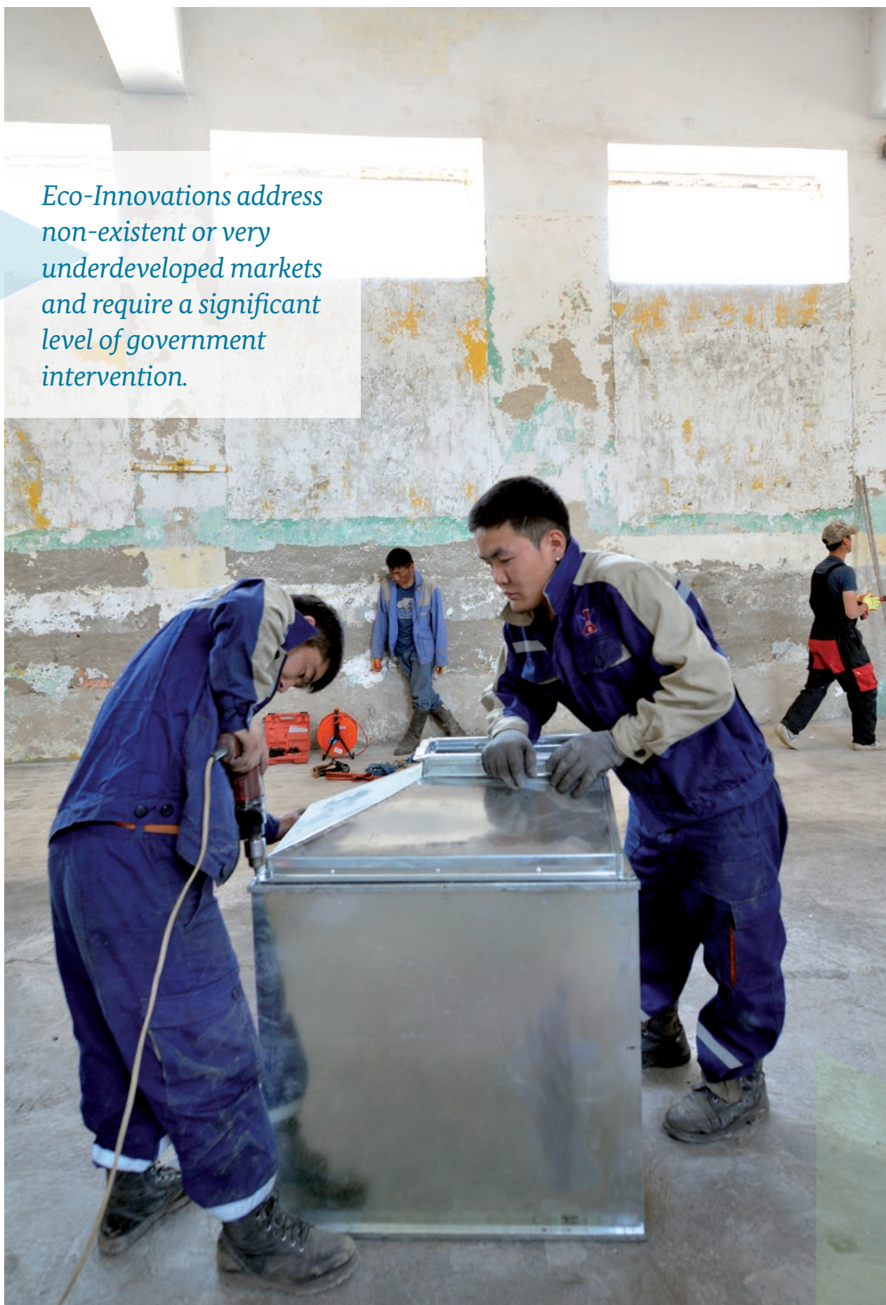
Thermal renovation of a school, Mongolia
