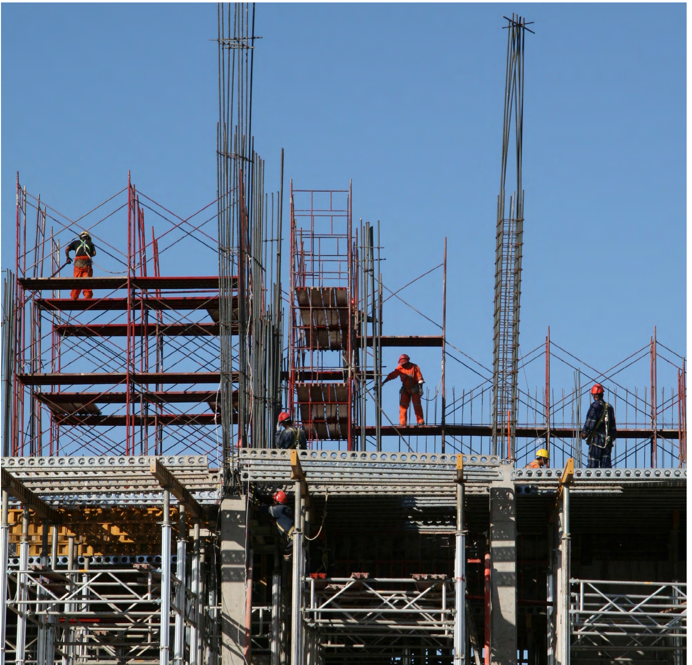
Construction site in Valdivia, Chile
