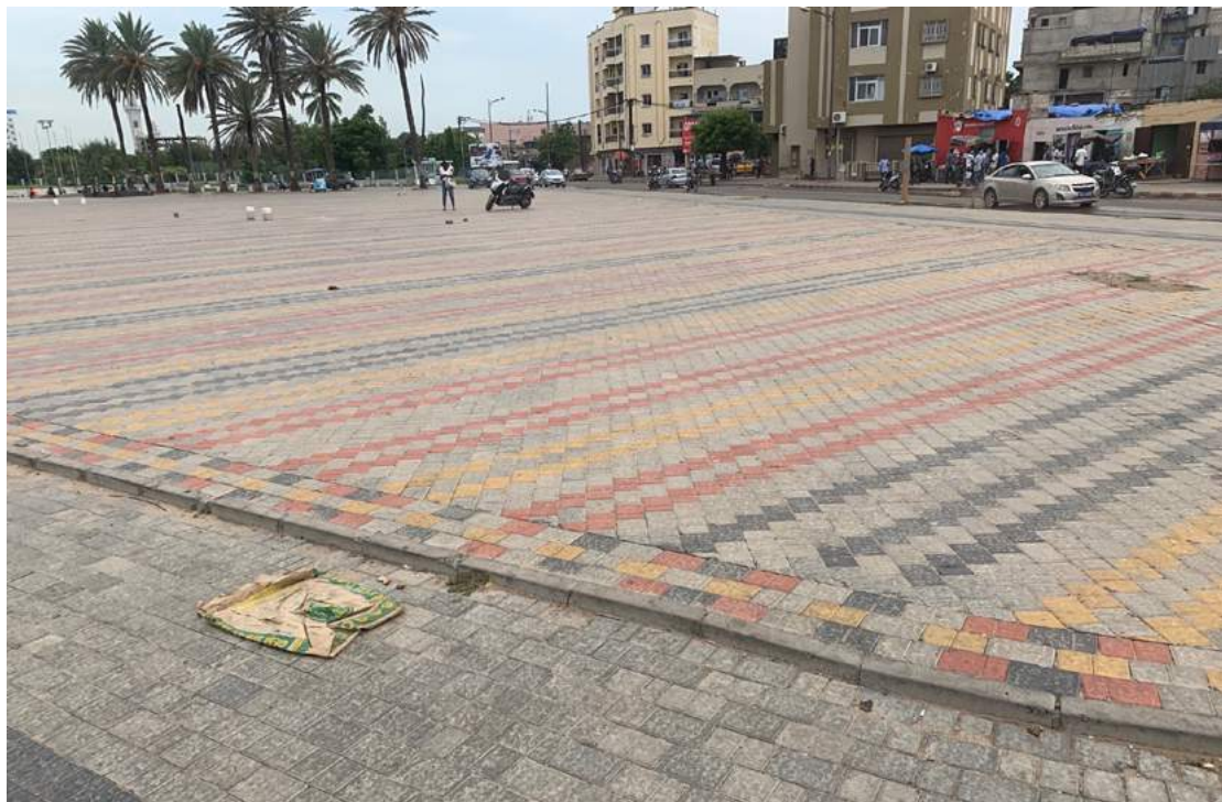
Figure 37: Paving stones from recycled material at Santenaire, Dakar
