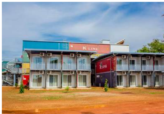
Figure 8: Back view of reused containers for training centre
