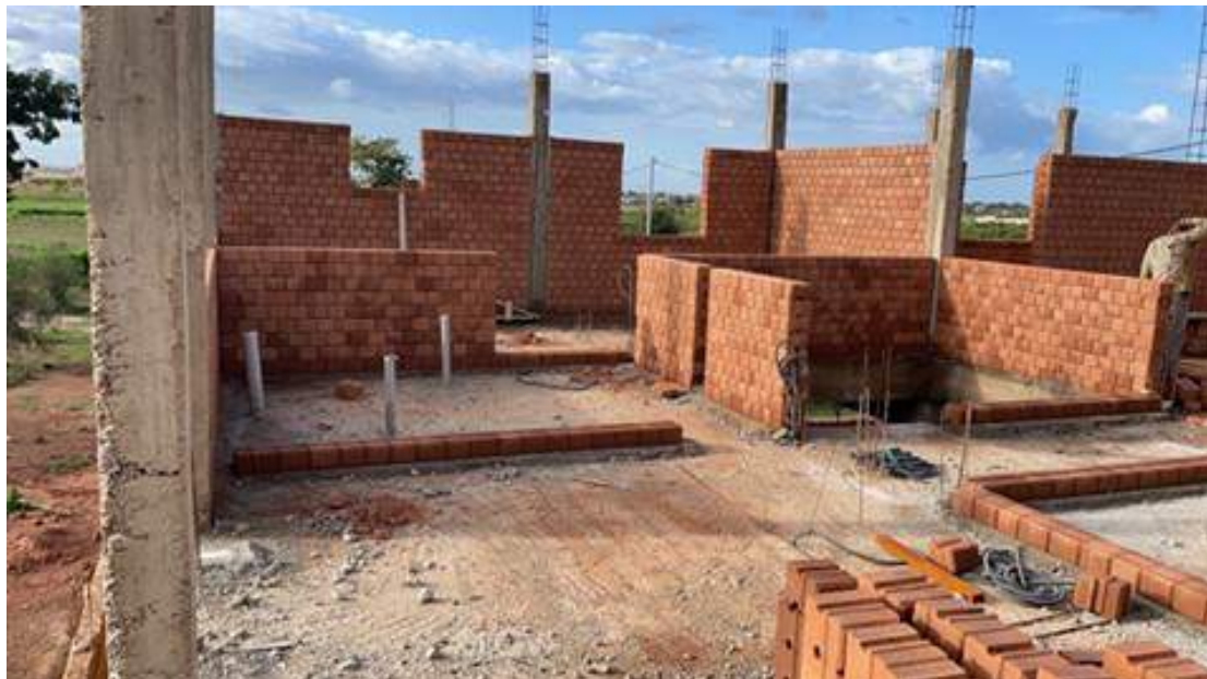
Figure 10: Construction project using CEB
