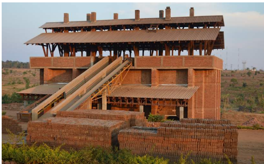
Figure 15: EcoKiln constructed in Malawi.
