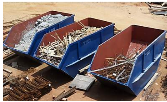
Figure 23: Sorting of construction waste on site
