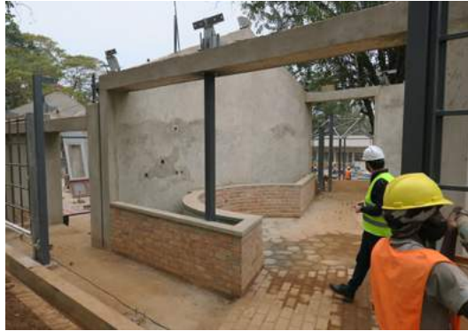
Figure 29: Old columns and structure maintained and strengthened
