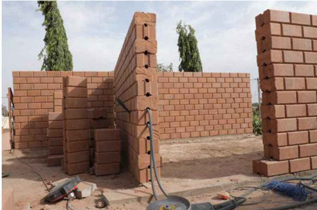
Figure 11: Zero waste interlocking CEB in construction
