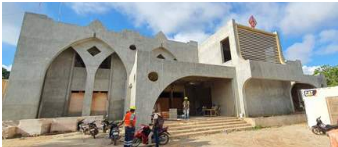
Figure 12: Newly refurbished Hotel Azalai
