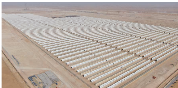
Dubai's concentrated solar thermal power plant
