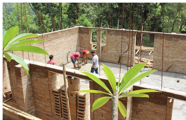
Photograph 9 House construction using CSEB. (Source: Build Up Nepal)
