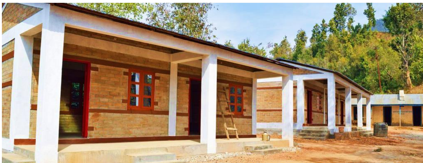
Photograph 10 Classrooms built with CSEB. (Source: Build Up Nepal)
