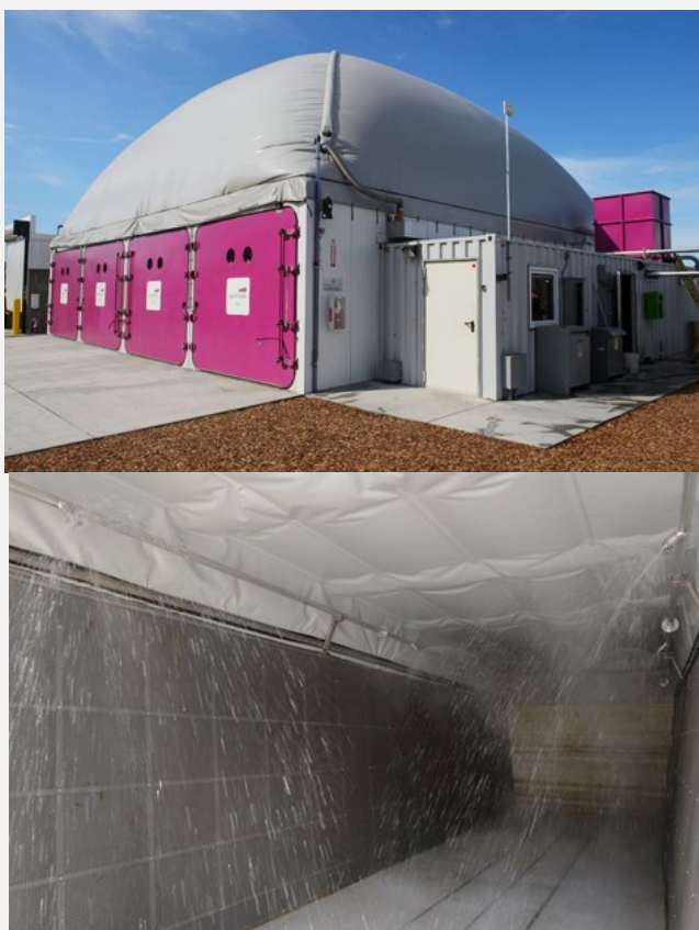
Smartferm Plug Flow Dry Anaerobic Digestion Technology, Monterey (U.S.) Image Source: Zero Waste Energy, 2013
