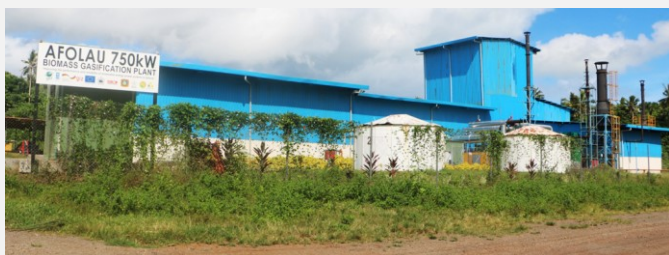
Afolau gasification plant in Samoa - commissioned Nov 2020 Image Source: UNDP, 2021
