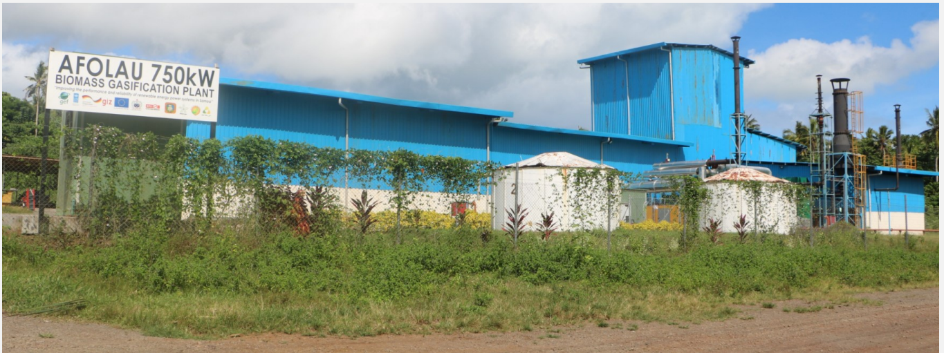
Figure 19 Afolau gasification plant commissioned Nov 2020
