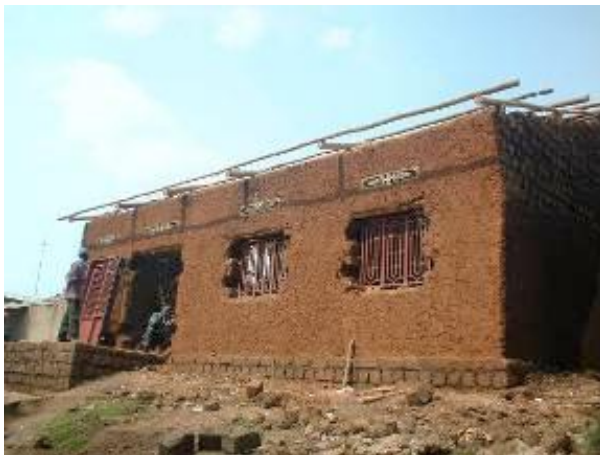
FIGURE 6-4 TRADITIONAL ADOBE HOUSE BEFORE PUTTING ROOFING
