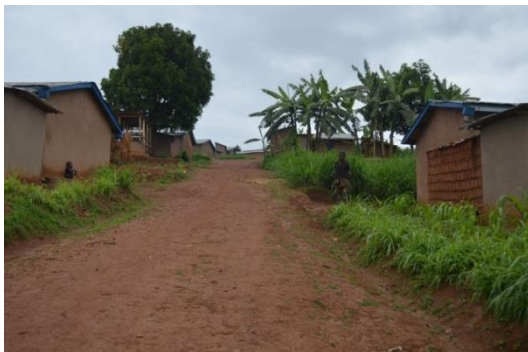
FIGURE 6-2 ACCESS ROAD ALONG THE SETTLEMENT
